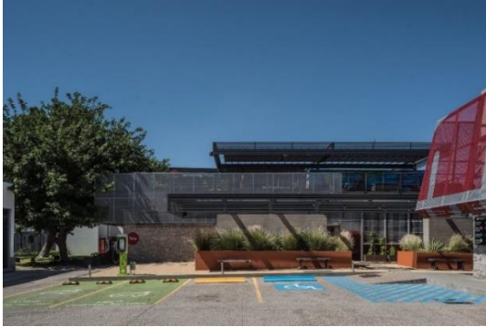
Figure 74 TERA BUILDING ALONG WITH PARKING (Arquitectos, 2015)
