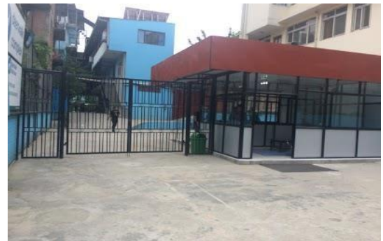
Figure 3-15 DWIT Entrance Gate
