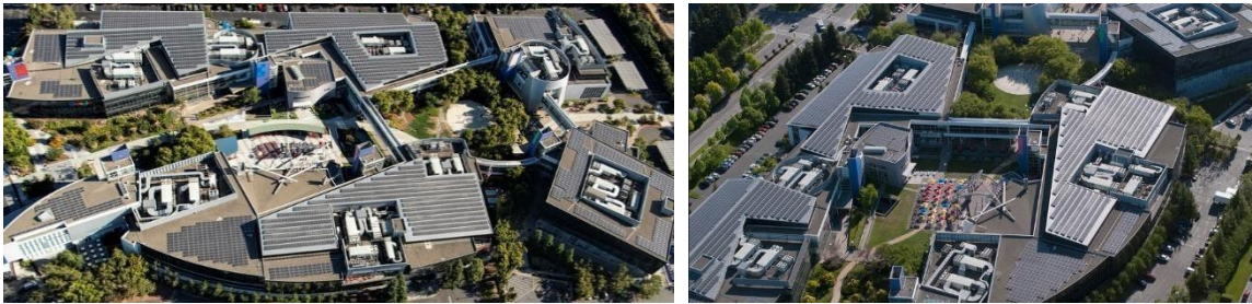
Figure 3-36 Solar Panels in roofing
