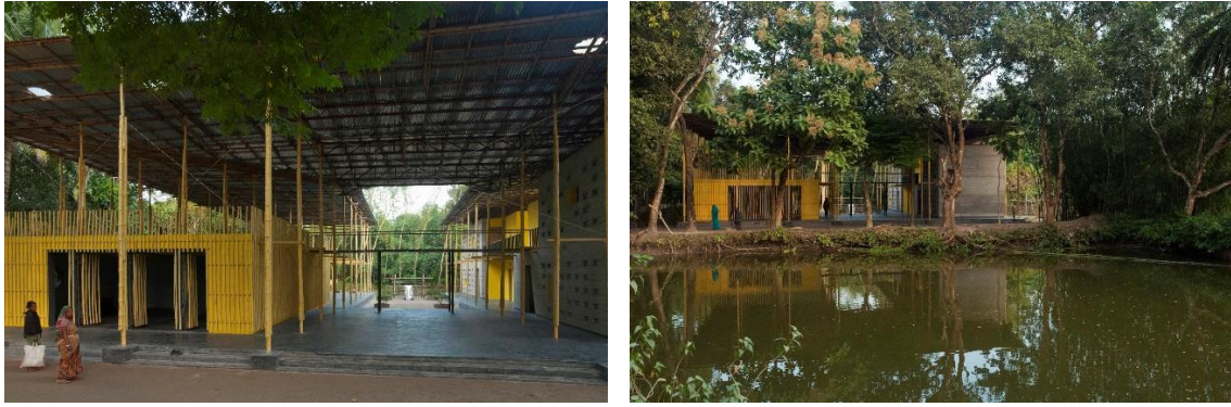
(a) (b) Figure 67 (a) Connecting Bridge (b) Nearby pond
