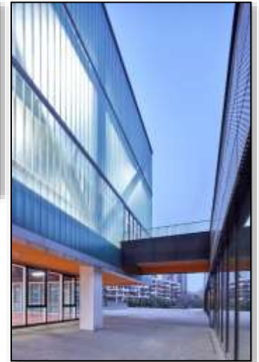
Figure 3.66 Bridge connecting stairs and multifunctional area
