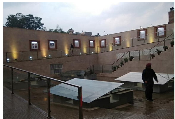
Figure 84: Ramp to the Gallery underneath the plaza, (Source: Ar. Abhishek M. Bajracharya)
