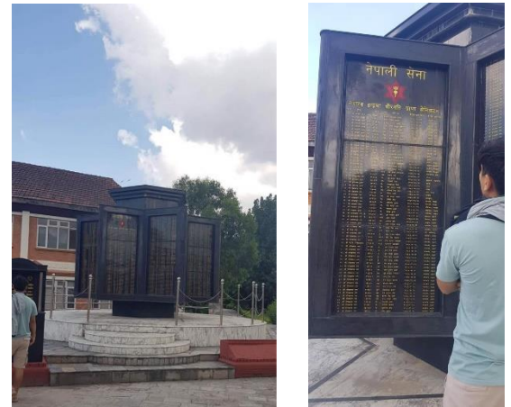
Figure 103: Sculpture in star shape with list of fallen soldiers with details of their postings and years (Source: Site study)
