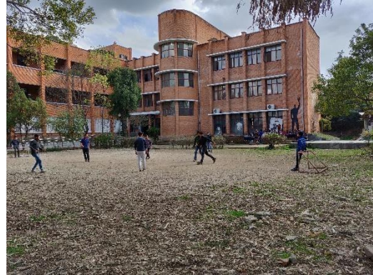
Figure 40: Architecture block, Pulchowk Campus
