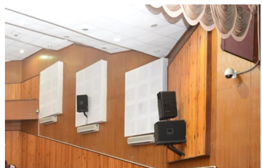
Figure 45: Projections in wall for proper sound diffusion as well as lighting system
