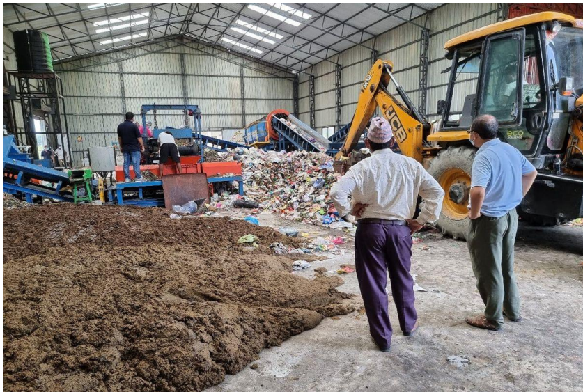
Figure 101: Organic waste being converted into energy
