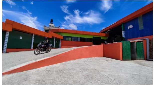
Figure 115: Existing Ramp on the site
