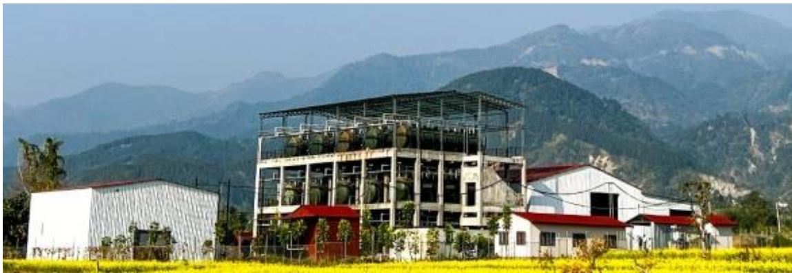
Figure 100: Waste to energy Plant in Dharan
