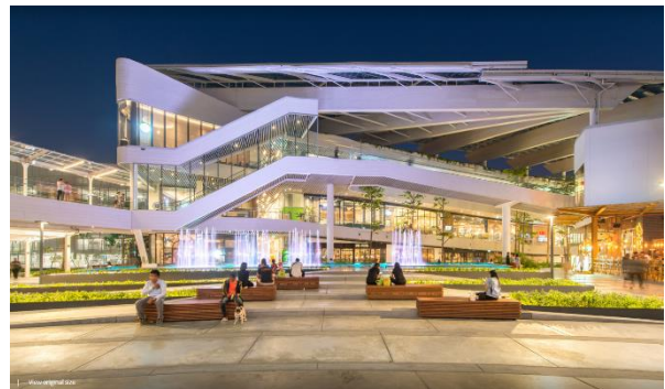
Figure 85: Exterior View of Mega Food Walk
