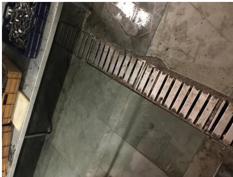
Figure 3-24: Use of drainage gullies in Kitchen
