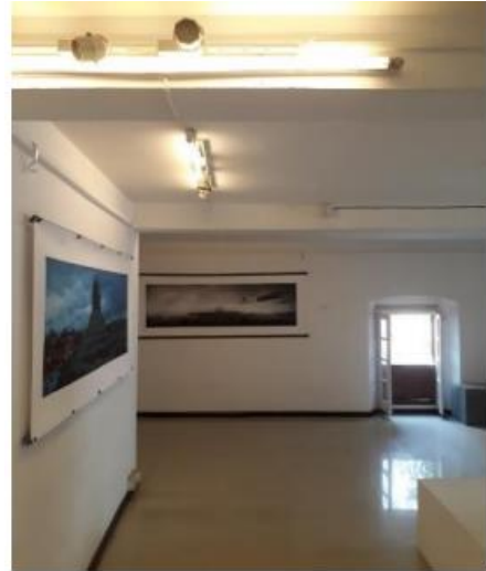
Figure 3-17 Artificial Flourescent tubelights and adjustable spotlights are used in upper gallery
