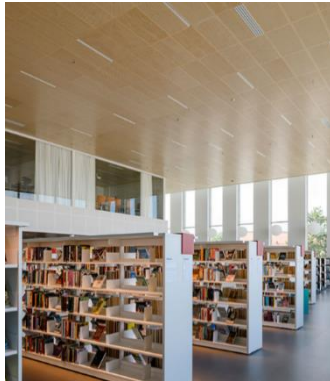
Figure 38: Acoustic wood wool ceiling, sustainable solution for acoustically outstanding spaces
