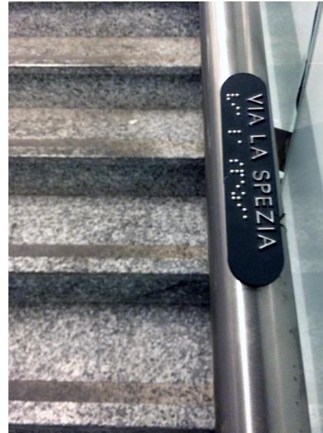
Figure 65: Example of Braille Handrails (Pigneto Metro Station, n.d.)
