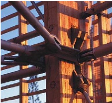
FIGURE 133 STEEL SUPPORT IT THE STRUCTURE
