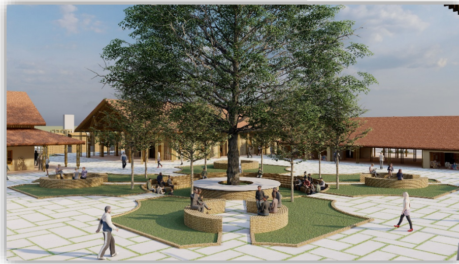
FIGURE 192 VIEW OF CHOWK
