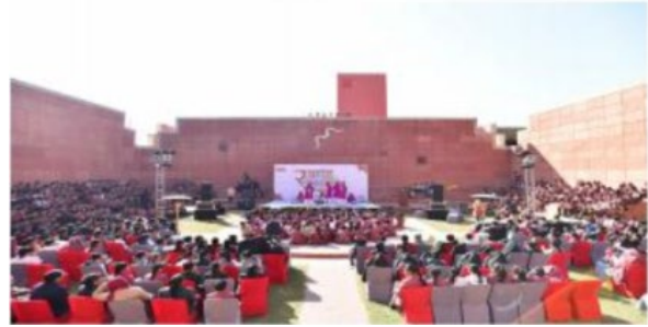
FIGURE 142 VIEW OF OPEN-AIR THEATRE
