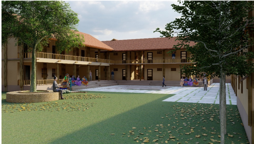
FIGURE 185 VIEW OF ACCOMMODATION BLOCK
