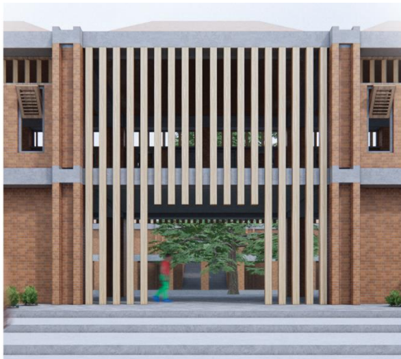
Figure 105 Battens as a prominent feature in the entry
