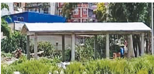
Figure 78 Unused pati and ghat
