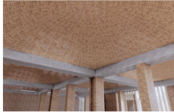
Figure 115 Rhotak dome from the inside
