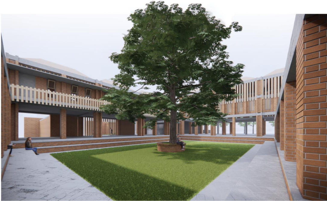
Figure 121 The main courtyard
