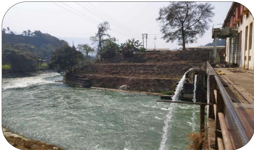
Figure 4.5: Tailrace diverging water into the main river stream (Sub-Basin No. 33)
