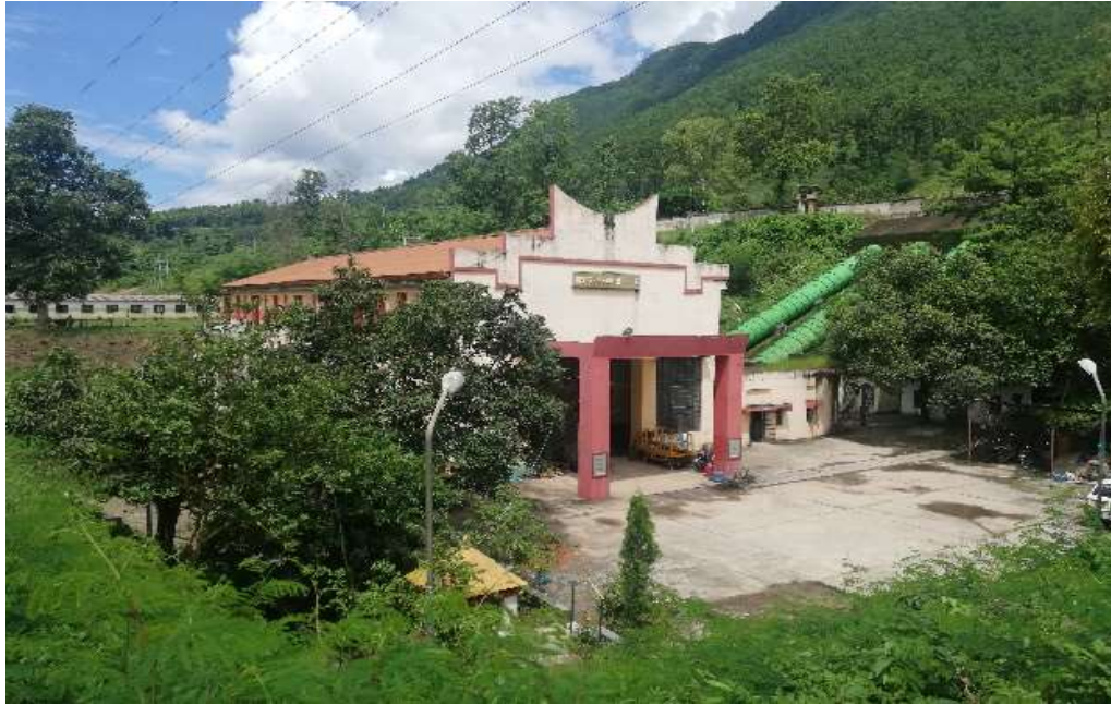
Figure 3.3: Devighat Hydropower Powerhouse with Sloping Penstock
