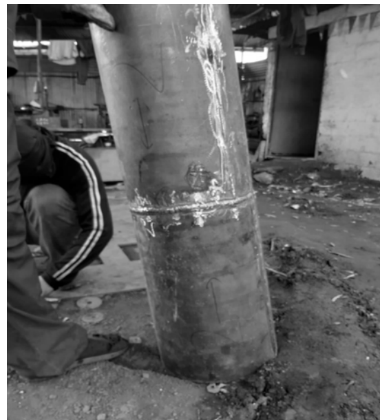
Figure 3.4: Welded prototype pipe shell
