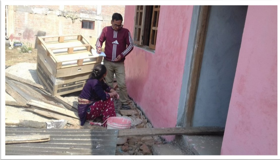
Photo 1 while doing questionnaire survey with the women mason working
