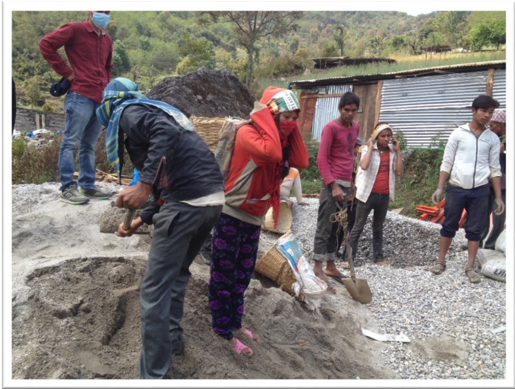
Photo 4 Women mason working in construction site
