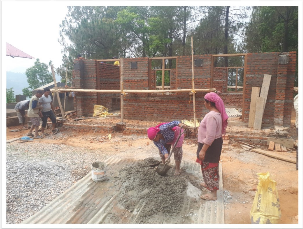
Photo 3 Women mason working in construction site
