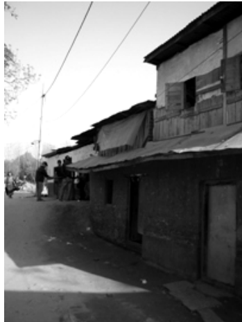
Figure 5.17: Connection of electricity in Banshighat, Kathmandu (2008)
