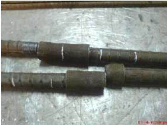
Photograph no 13: Thread slip failure and failure due to breaking of coupler
