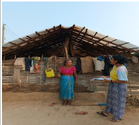
Figure 4. House damaged by elephant
