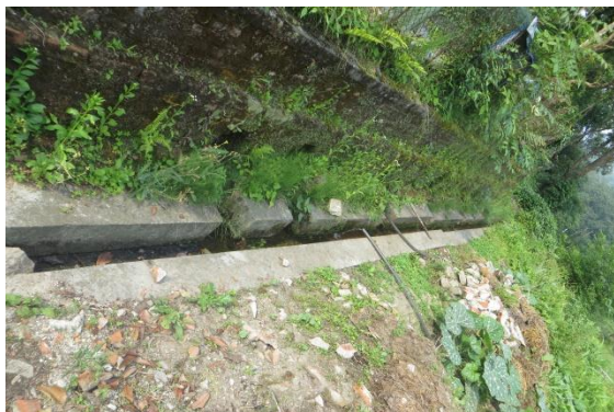
Water collected from different source using pipe lines.
