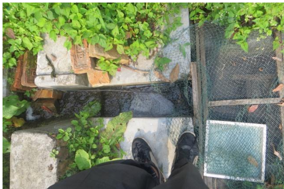
Water filtered using net to stop leaves into water reservoir
