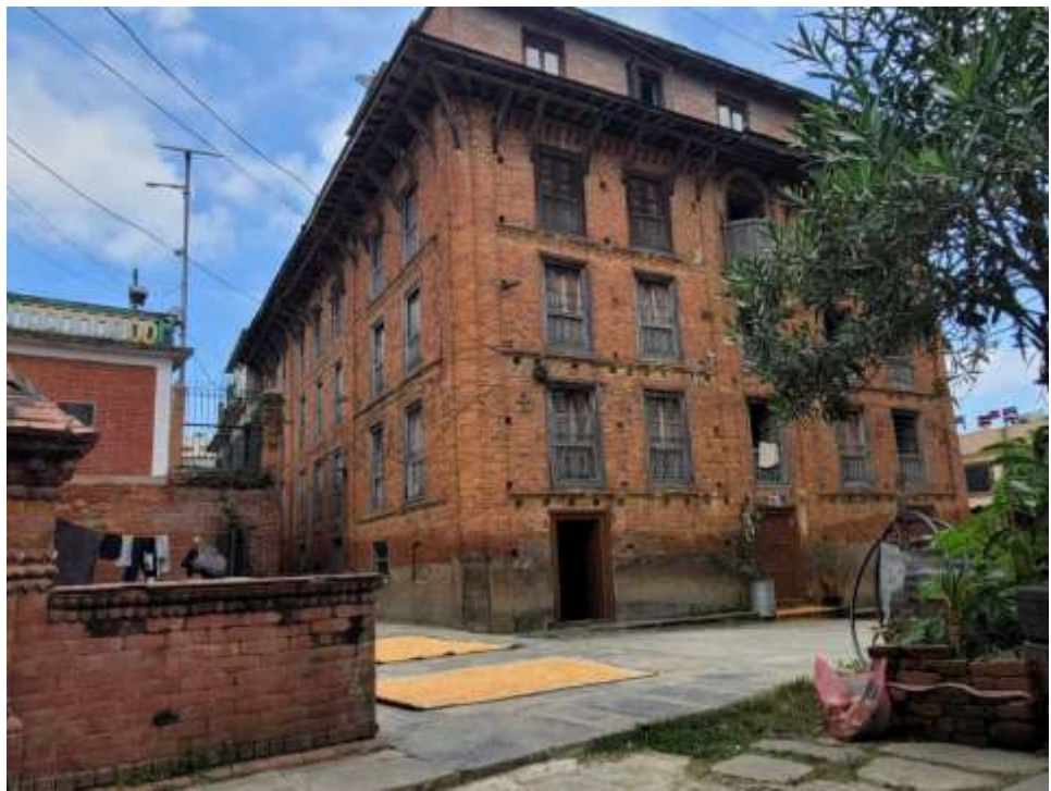
Photo 28: Unique Newa architecture private building at Chochen
