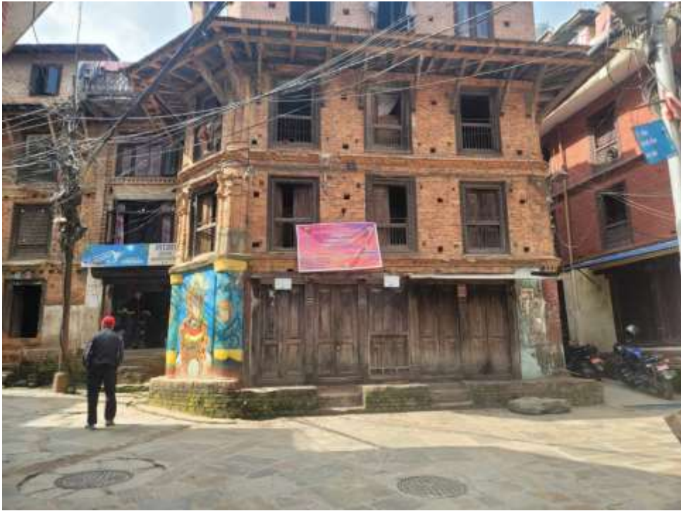
Photo 27: Unique Newa architecture private building at Chapachhen
