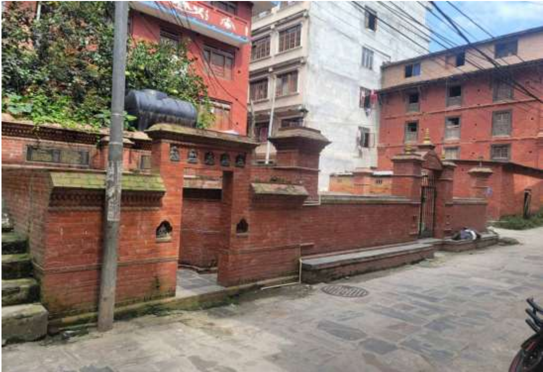
Photo 25: Concretisation of Siddha Pokhari
