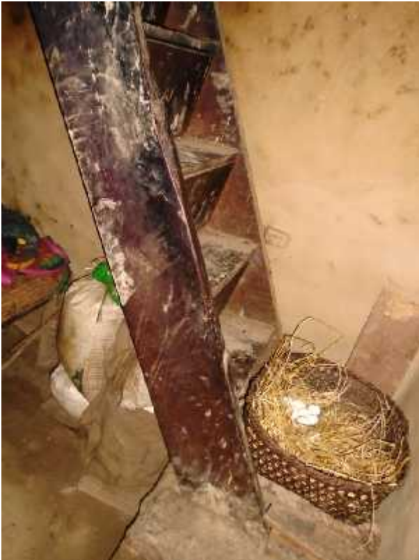
Staircase leads first floor (photo: Milan Bagale/field study, 2015)
