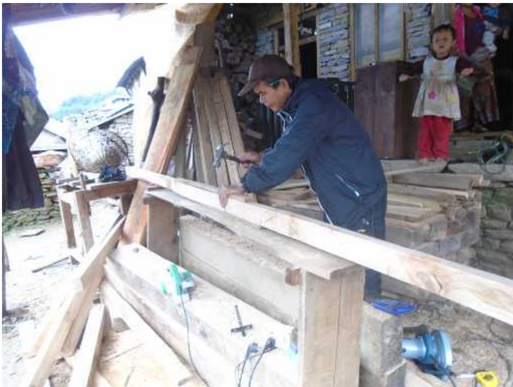
Mr. Balaram Gurung preparing wooden frame (photo: Milan Bagale/field study, 2015)
