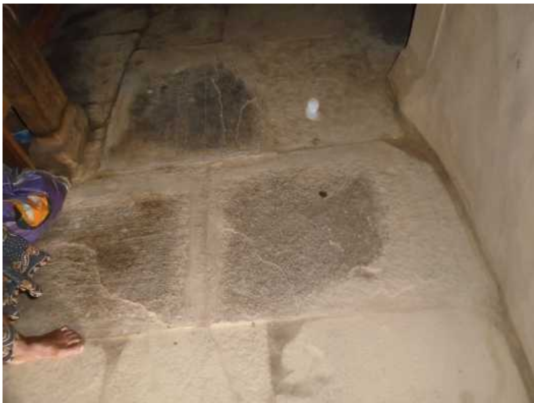
Stone as a flooring material in kitchen (photo: Milan Bagale/field study, 2015)
