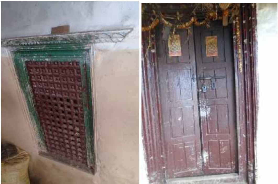
Door-Window Detail (photo: Milan Bagale/field study, 2015)
