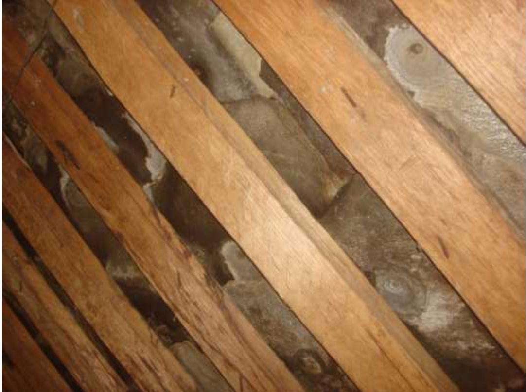
Slate fixing detail (photo: Milan Bagale/field study, 2015)
