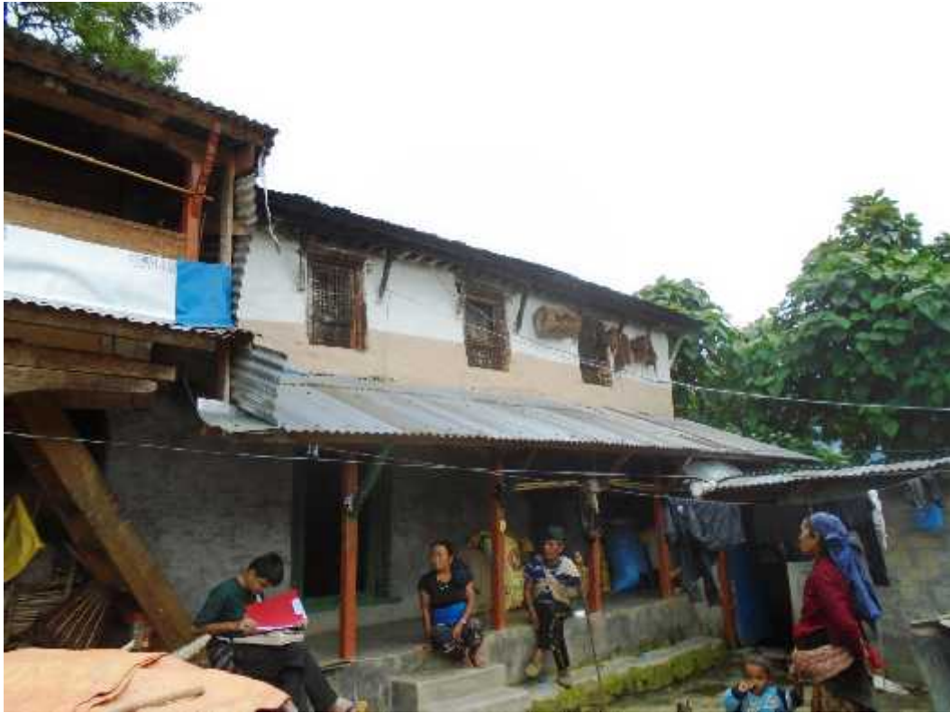
Building owned by Maya Devi Gurung (photo: Ram Shrestha/field study, 2015)
