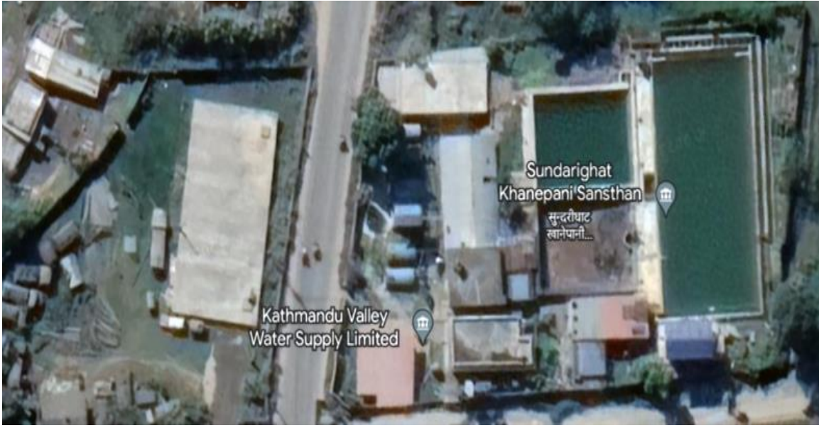
Figure 8: Sundarighat water treatment plant
