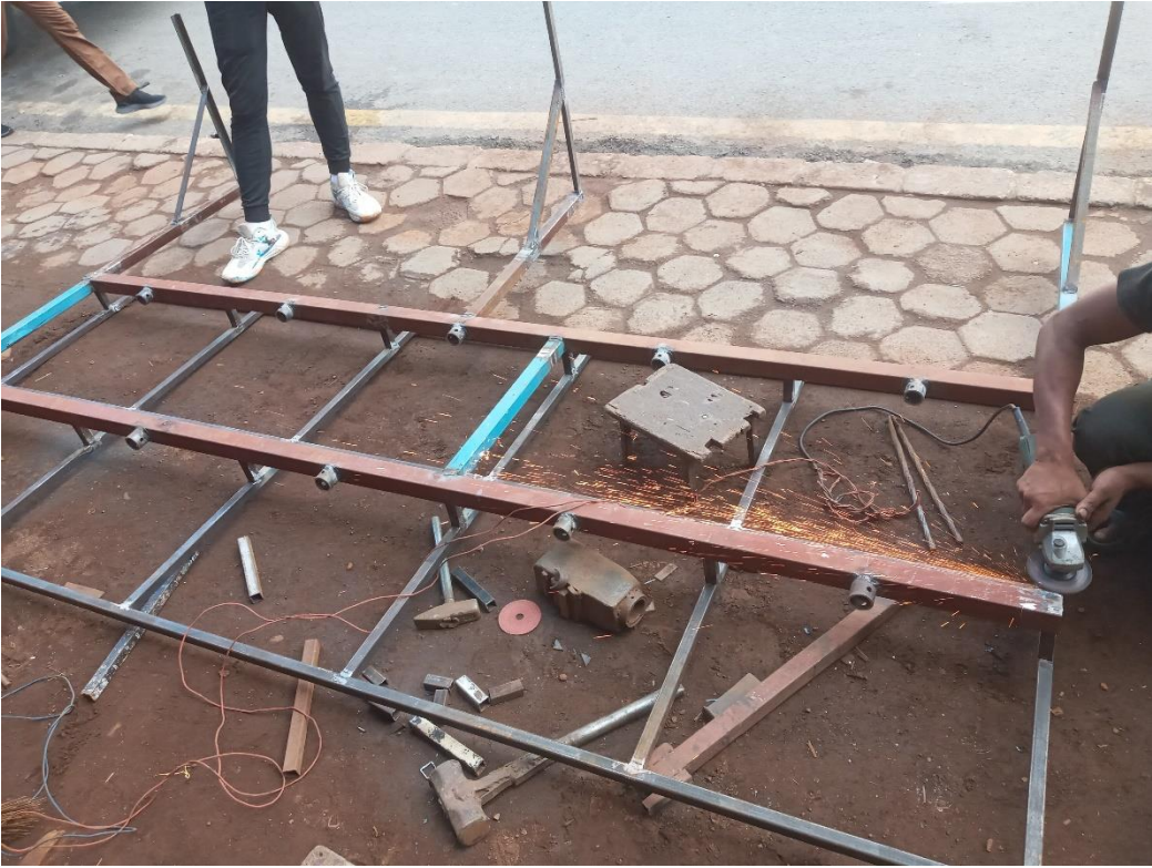
Figure 42 Fabrication of Frame to hold Multiple Fan
