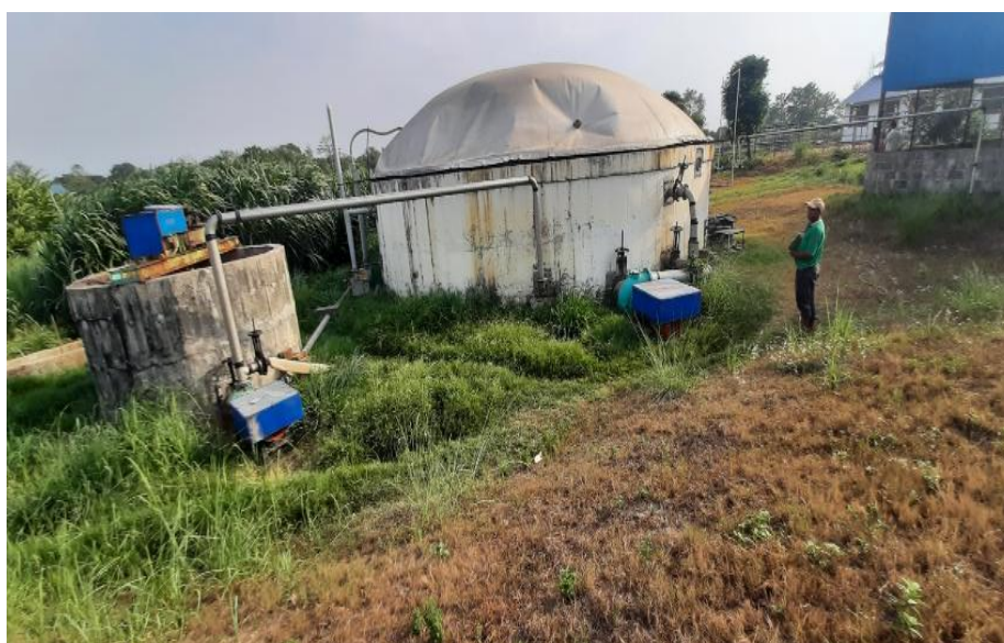
Figure 5: Site Location at Rampur, Chitwan
