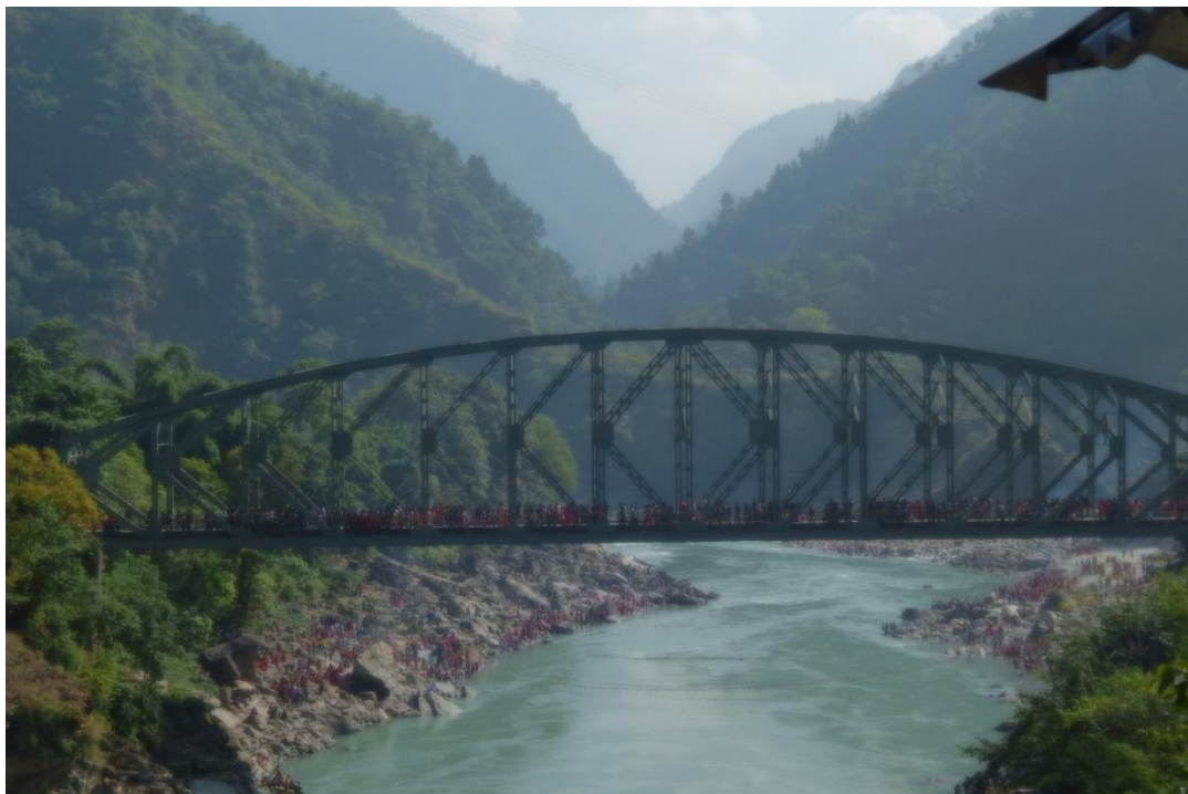
Ramdi Bridge joining Palpa and Syangja District at Siddhartha Highway
