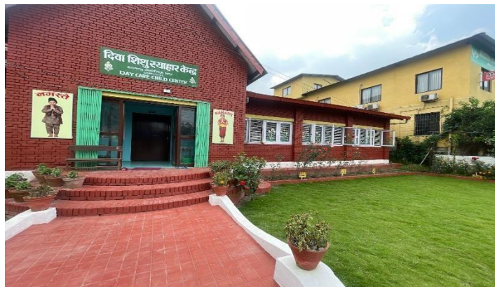
Figure 50 Diba Child care centre inside Industrial area
