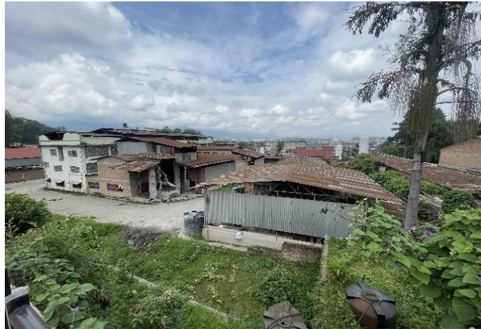
Figure 44 Side view of industrial Infrastructure (Building) from community
