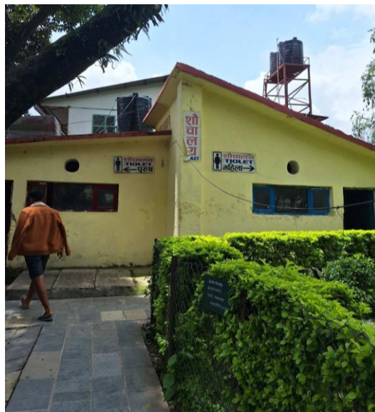
Figure 18 Toilet present in Park
