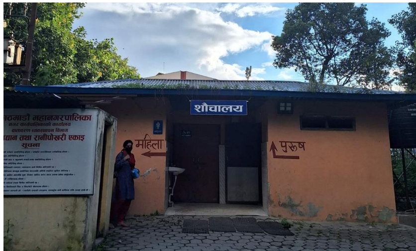
Figure 30 Toilet in the Park
