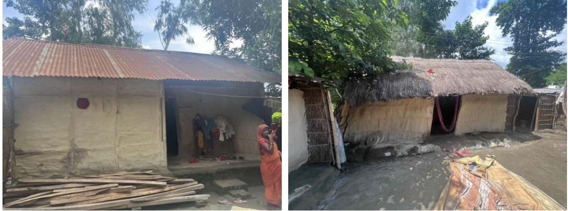
Figure 22: Condition of Houses at present
