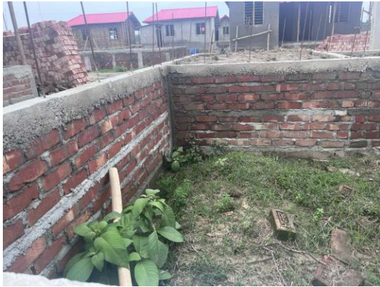
Figure 38: Raised Plinth levels
