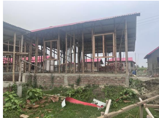
Figure 39: Bamboo Frame structure
