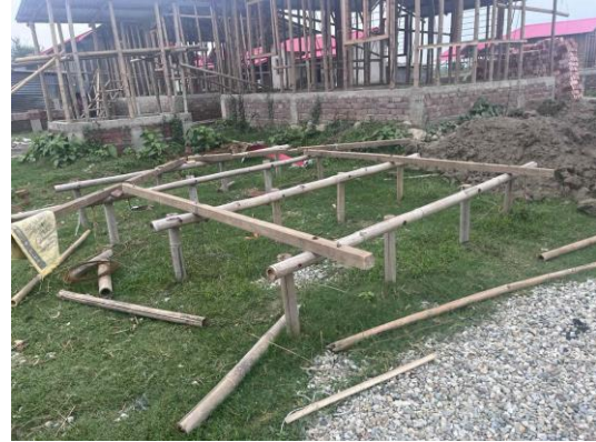
Figure 37: Platform of bamboo raised for plinth
