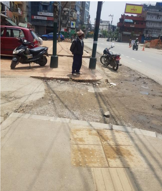
Figure 4.2 Footpath section at chainage 0+400 to chainage 0+500 (left side)
