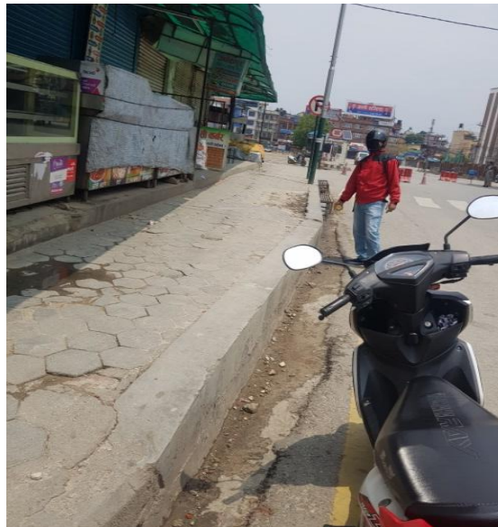
Footpath section at chainage 1+300 to chainage 1+400 (left side)
