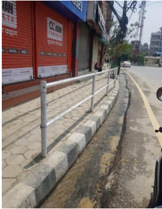
Figure 4.3 footpath section at chainage 1+600 to chainage 1+700 (left side)
