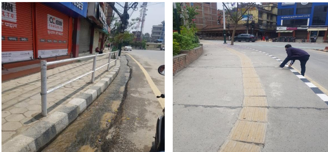
footpath section at chainage 1+600 to chainage 1+700 and 0+000 to chainage 0+800 (left side)
