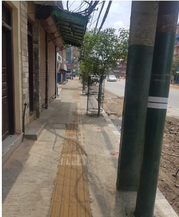
Figure 4.1 footpath section at chainage 0+200 to chainage 0+300 (left side)
