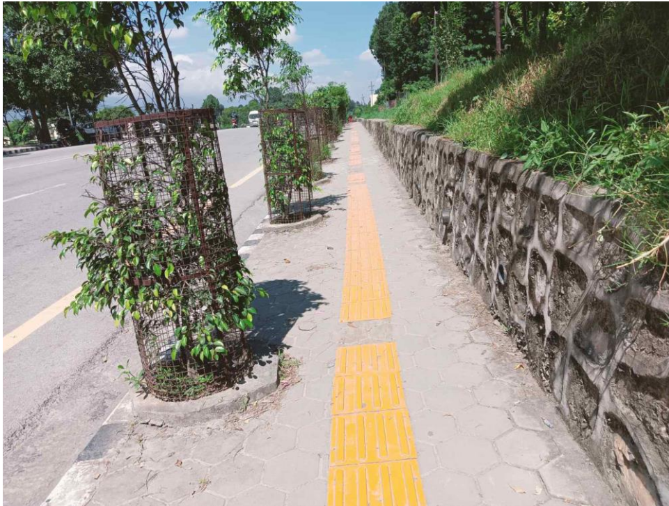
Figure3. 11: Sidewalk along with Tactile pavement along Sanothimi Road
