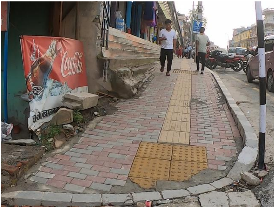
Figure3. 8: Side Walk along with Tactile Pavement along Jorpati Road
