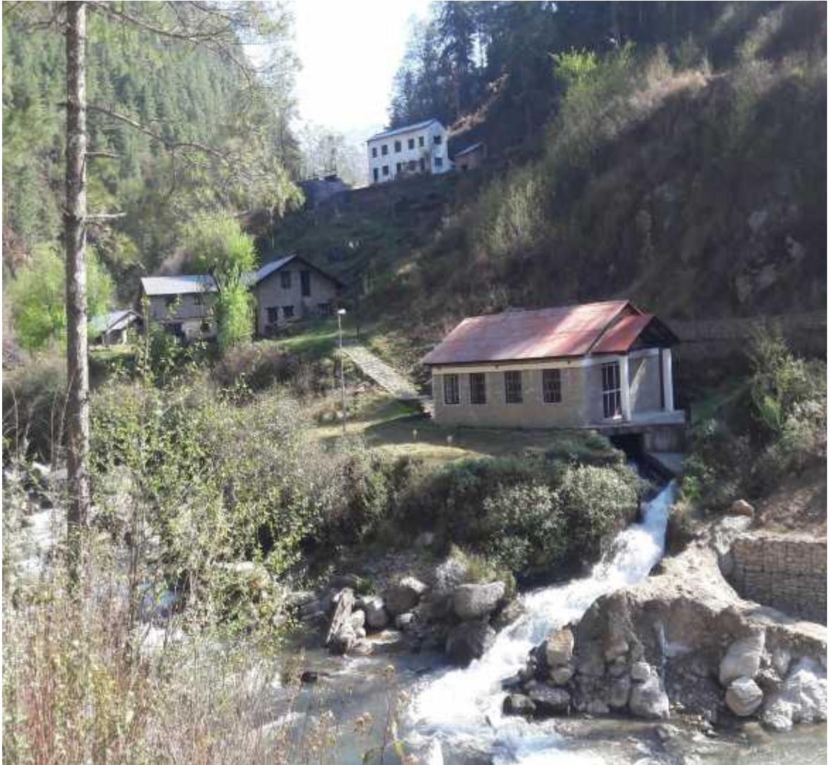
Power House site Salleri Chialsa Electricity Company Limited
