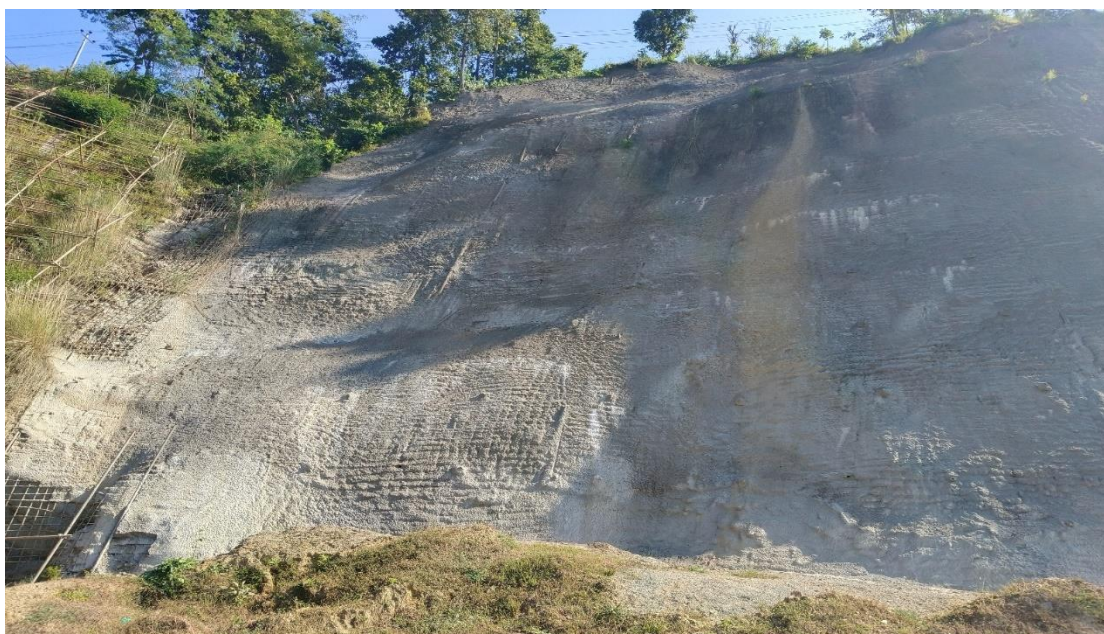
Figure 2-1 Soil Nailing works being done at Pasang Lambhu Highway
