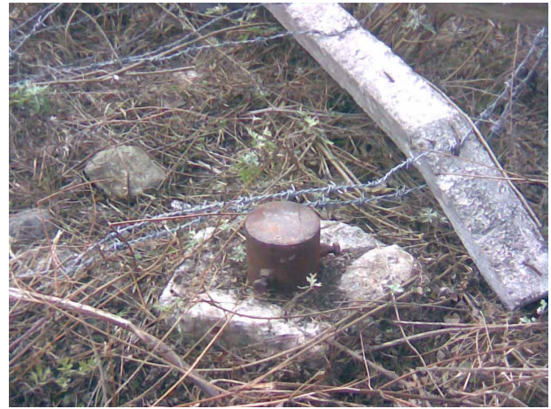
Plate 10: Bore hole-2 made for monitoring groundwater quality near leachate tank of valley 2
