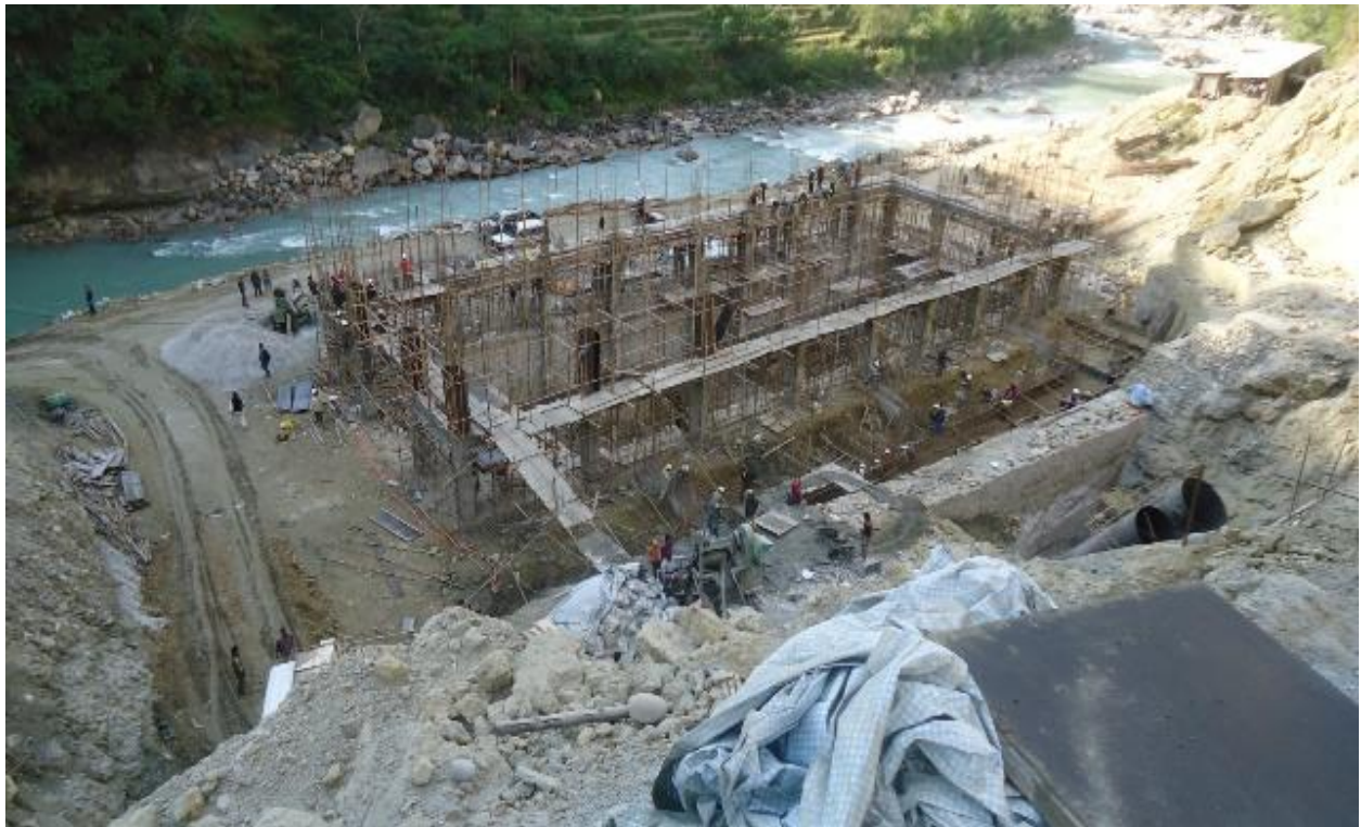
Photograph 9: Construction site of Modi Hydro Power Parbat (10 MW) financed by CEDB.
