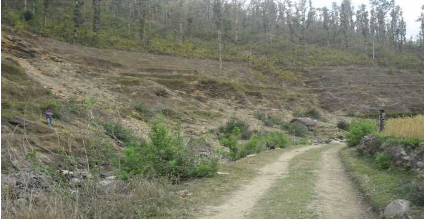
Picture1: Before Construction of Tiperi Khola bridge over Tiperi khola, Dailekh
