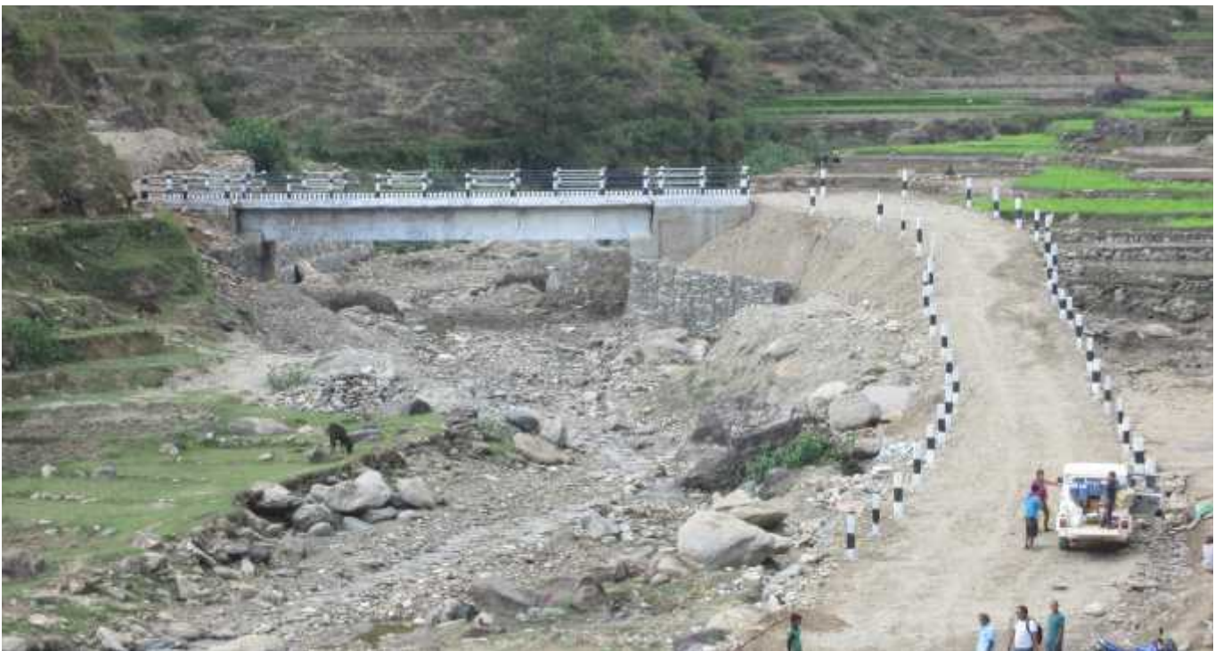
Picture 2: After construction of Tiperi Khola Bridge over Tiperi khola, Dailekh
