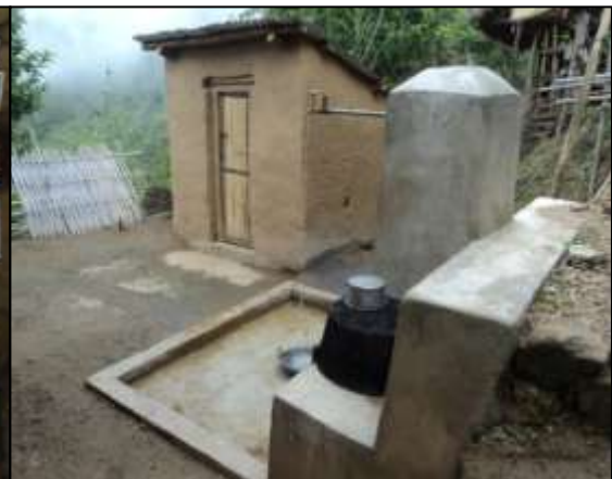
Infrastructure done by co member
