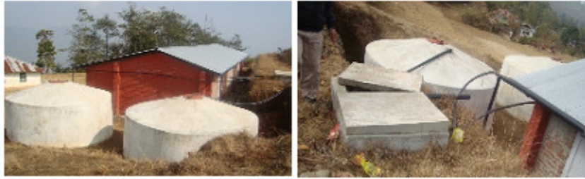
Rain water harvesting system
