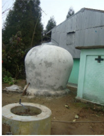
Figure 6: View of RWH jar along with Toilet attached Biogas Plant
