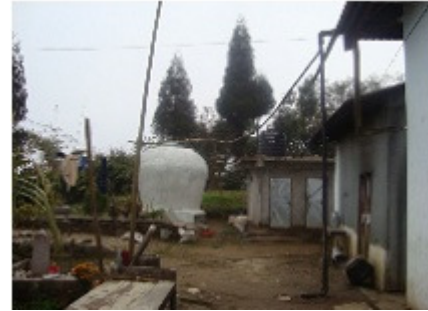
Figure 11:View of RWH System
