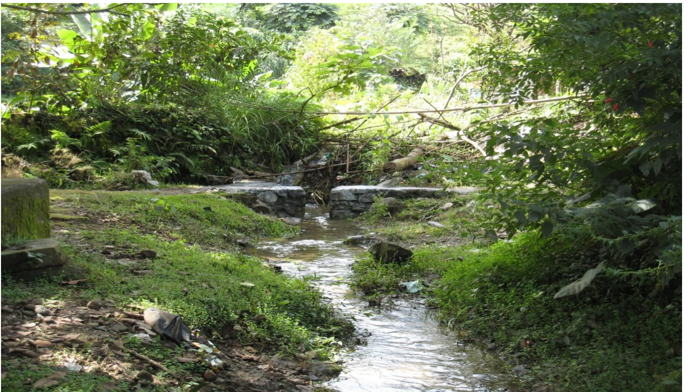
Main and Branch Canal
