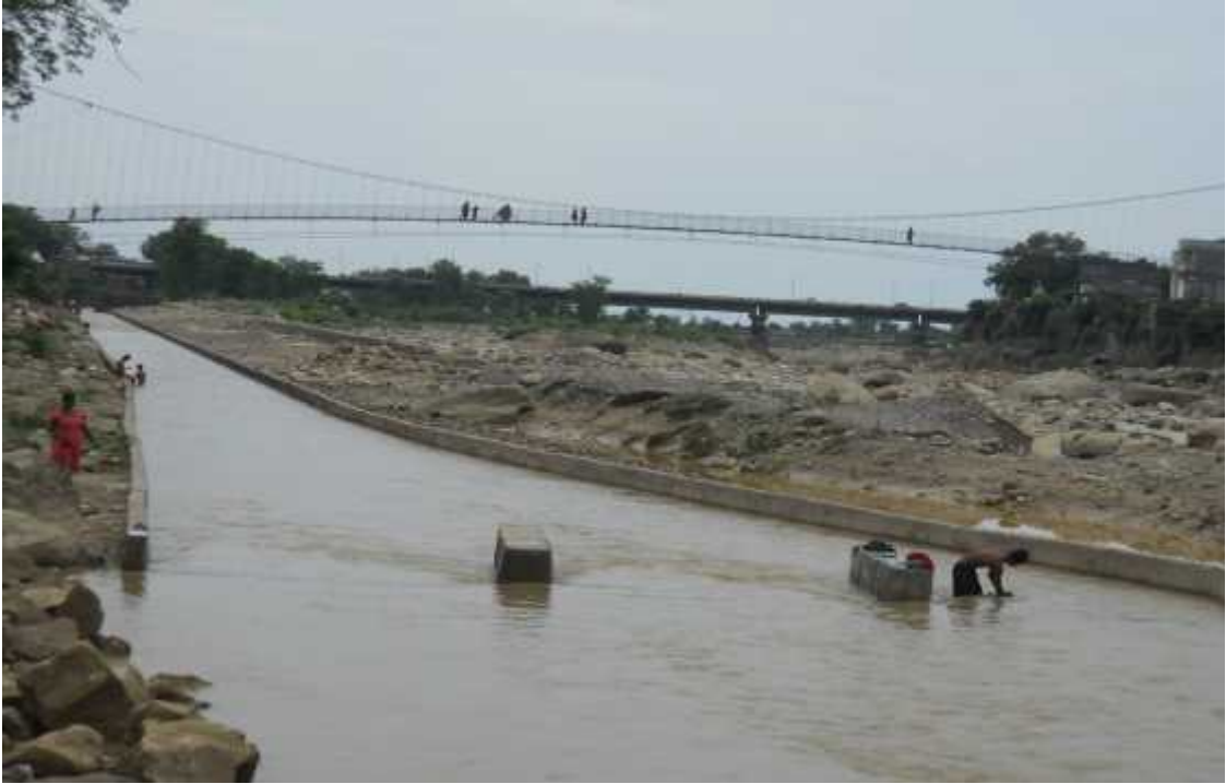
Origin of the system located in Butwal
