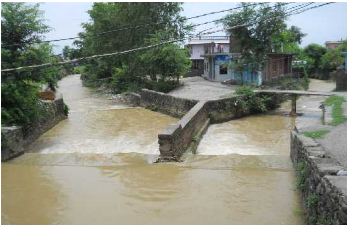
Water distribution Site of the System, Ittabhod
