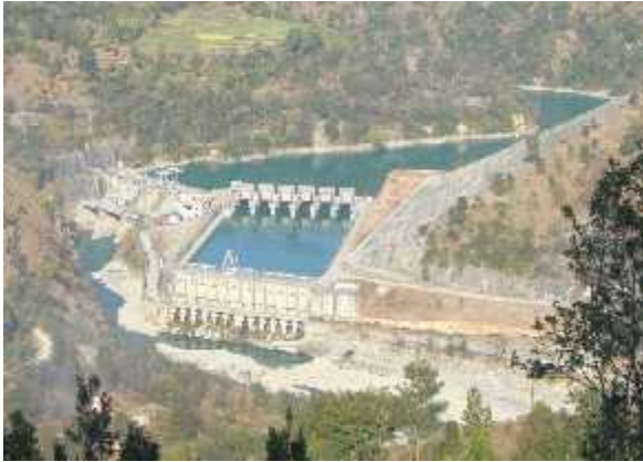
Kaligandaki Hydro-power dam (Study area).
