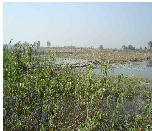
Jagdishpur Reservoir (north face close to inlet)
