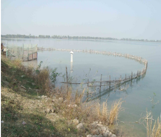
Jagdishpur Reservoir (south face near main outlet)
