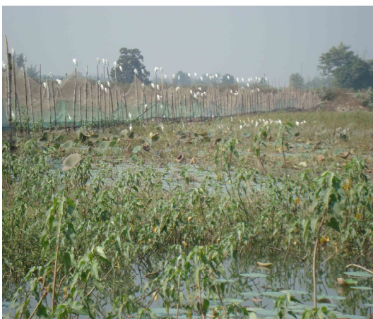
Jagdishpur Reservoir (north face close to inlet)
