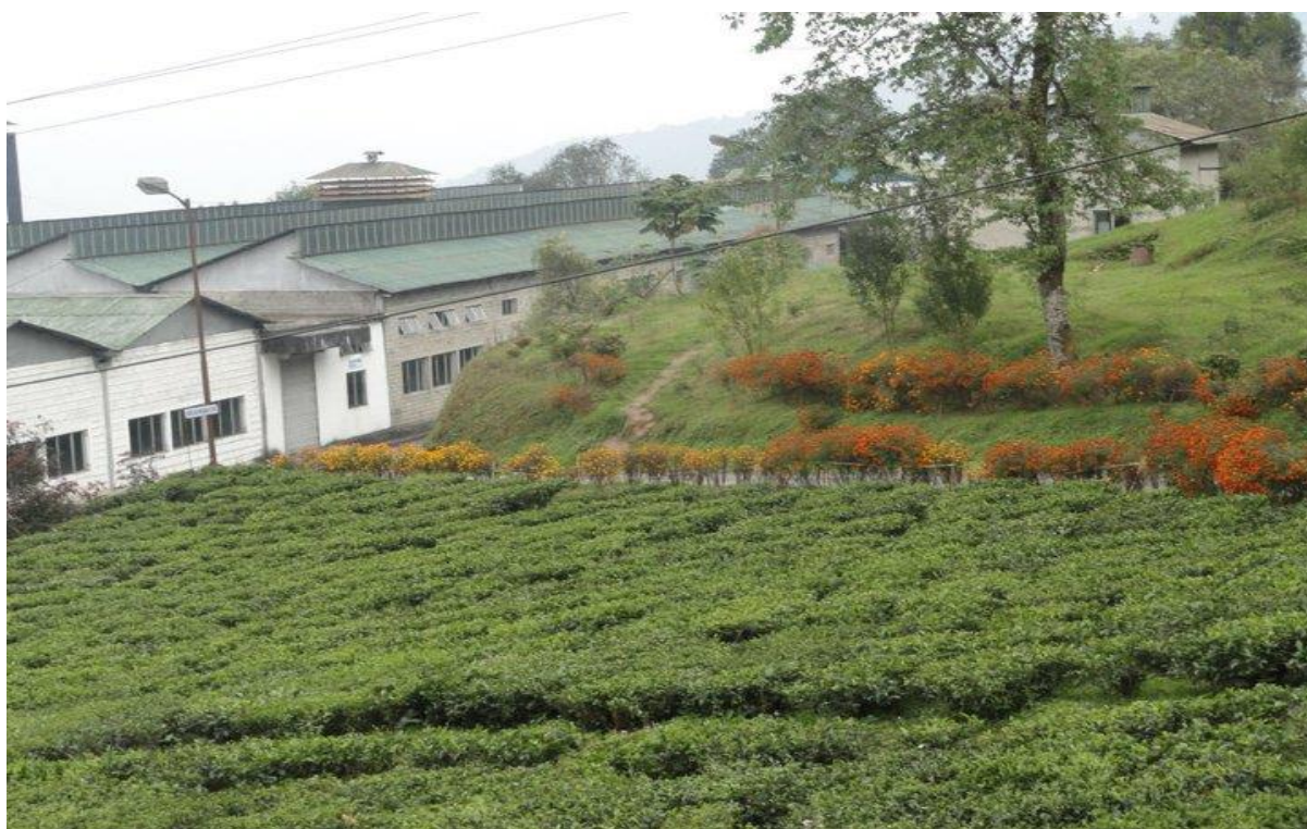
A Side View of Temi Tea Estate Factory.
