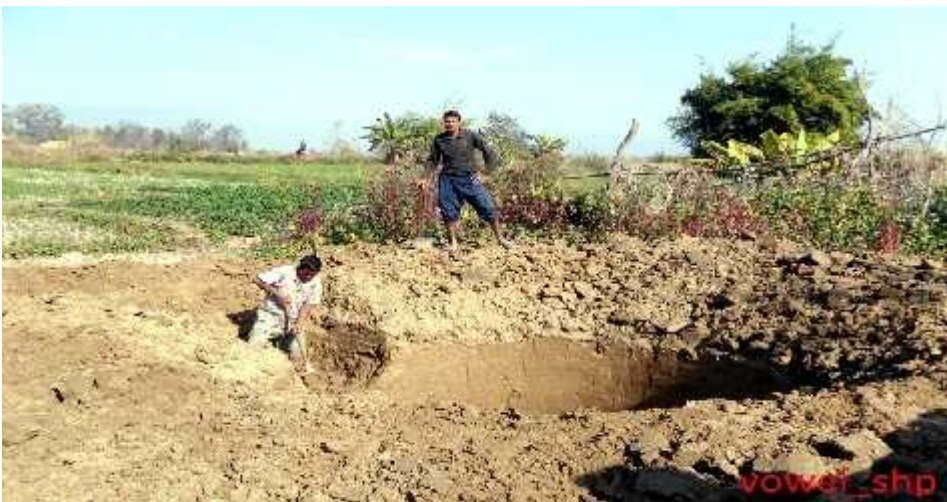
Picture -6 Biogas plant under construction with the support of Chandanpur CFUG
