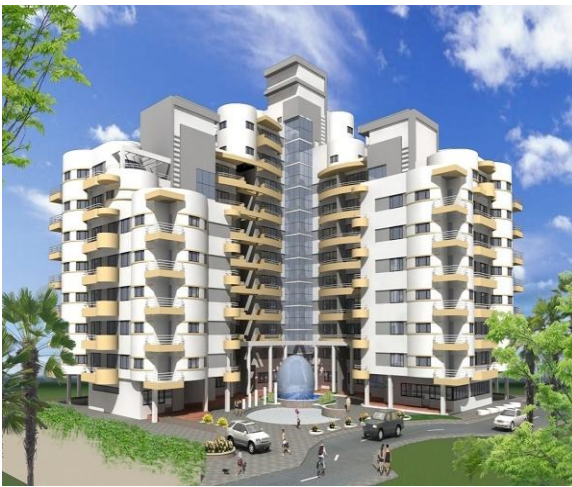
Figure 1: 13 Stories Apartment Building At Sundhara, Kathmandu (Under construction)
