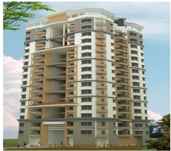
Figure 2: 18 stories Apartment Building at Dhapakhel, Lalitpur, (Under construction)
