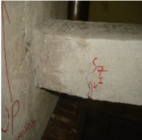
Progression of flexural crack Specimen, S7
