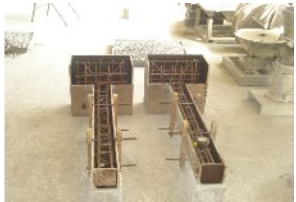
Fig.3, Rebar cage inside Form and clamping of form
