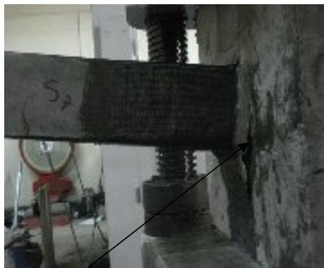
Crack at joint
