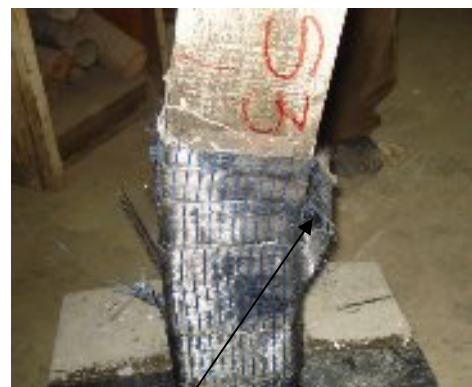
Delaminating of CFRP
