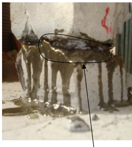
Fig. 7.2. Epoxy grouting in cracks
