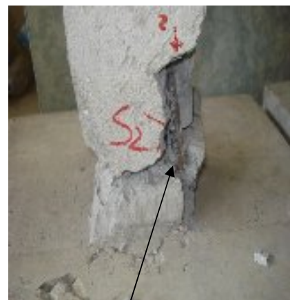
Damage seen after rupture of Reinforcement. Specimen. S2
