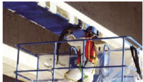
Application of U-wraps
