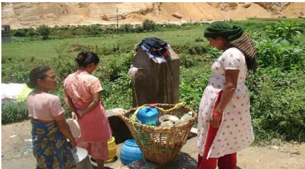
Photo - 2: A Community Tap, in the position of daily use by the community people
