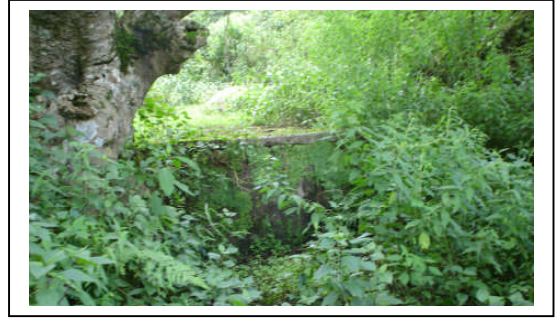
Spring Water Tank, Ward No. 8
