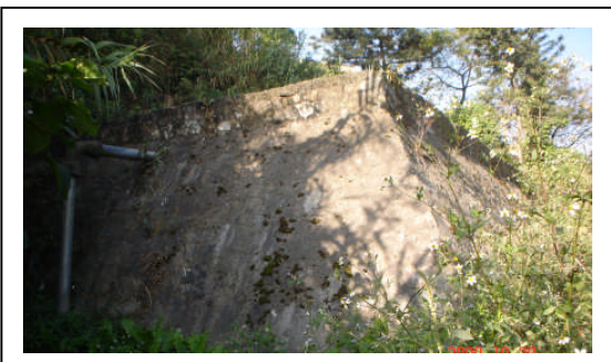
Reservoir, Ward No. 2
