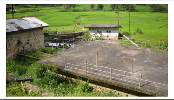
Reservoir, Ward No.7
