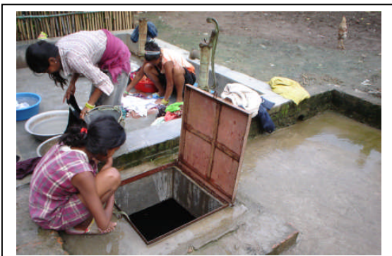
Rain Water Harvesting Tank, Ward No. 6
