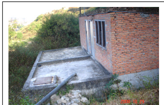
Reservoir, Ward No. 6
