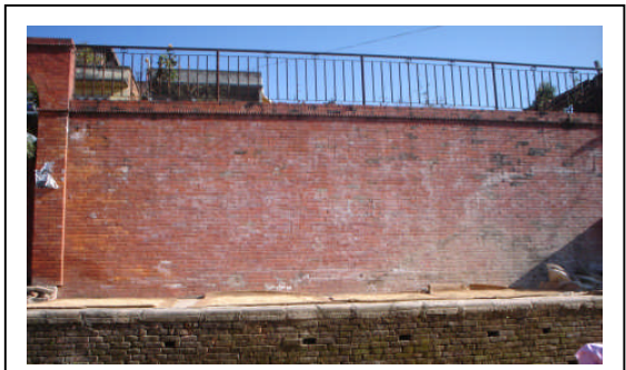
Reservoir, Ward No. 1
