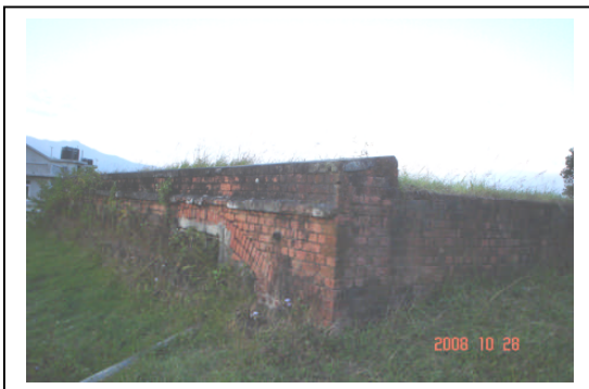
Reservoir, Ward No. 18
